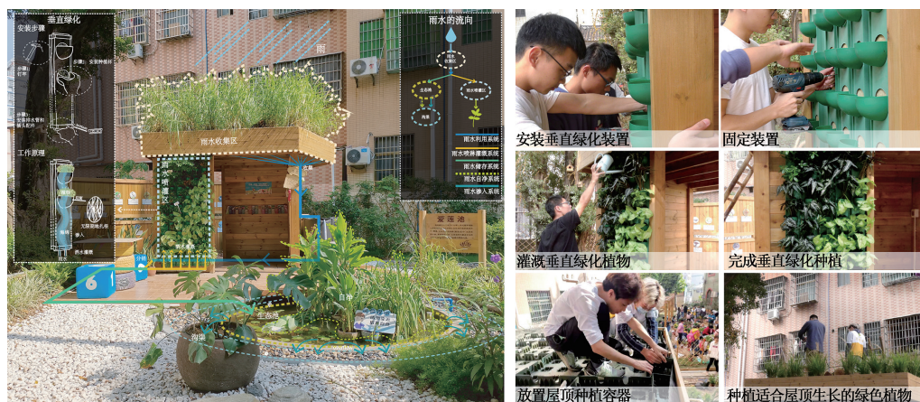
图3 立体绿化与雨水收集系统的搭建 Fig.3 Construction of three-dimensional greening and rainwater harvesting system
