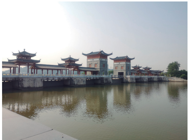
图9 长洲岛新担涌闸桥 Fig.9 The lock and bridge at Santan River on Changzhou Island
